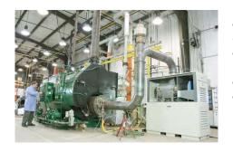
Researchers are developing a costeffective supplemental burner, integrated with a gas-turbine-based combined heat-and-power system. Laboratory tests have shown total efficiency of over 85% and NO<sub>X</sub> emissions that are below stringent California emission levels. Field testing is planned at a food-processing plant in California.
